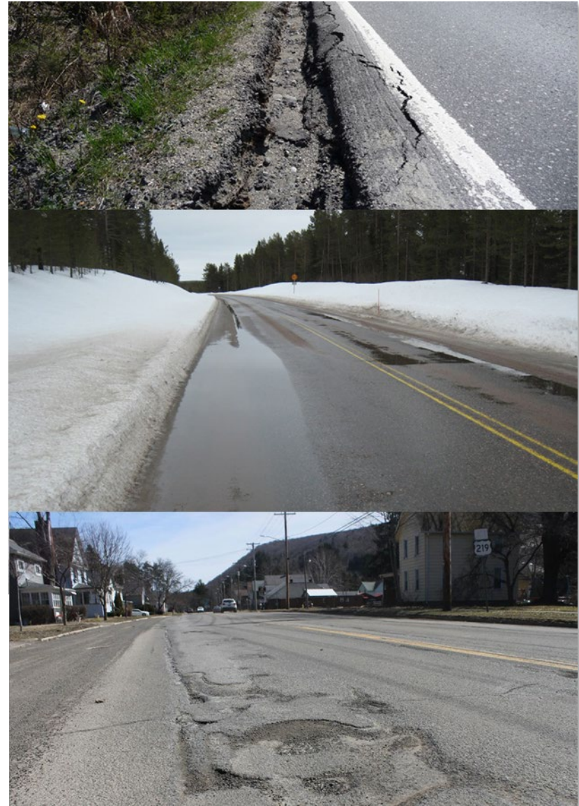
COMMON ROADWAY DRAINAGE ISSUES
